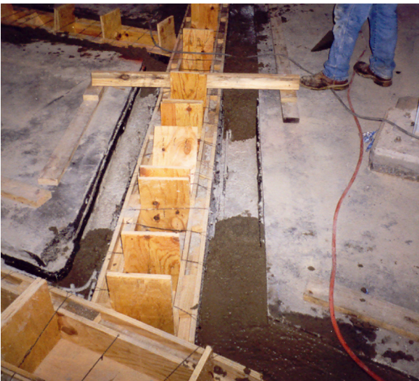
10. Sand bags are removed before the second lift of concrete is installed. The sand bags are no longer necessary, because the first lift of concrete has locked the liner in place, so it won't float.
