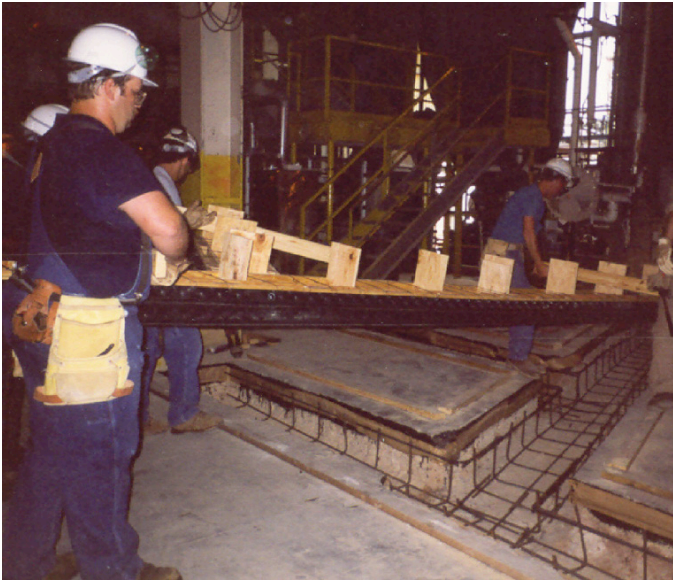
5. Workers carry the trench liners into the construction area by the 2 x 4 cross beams.
