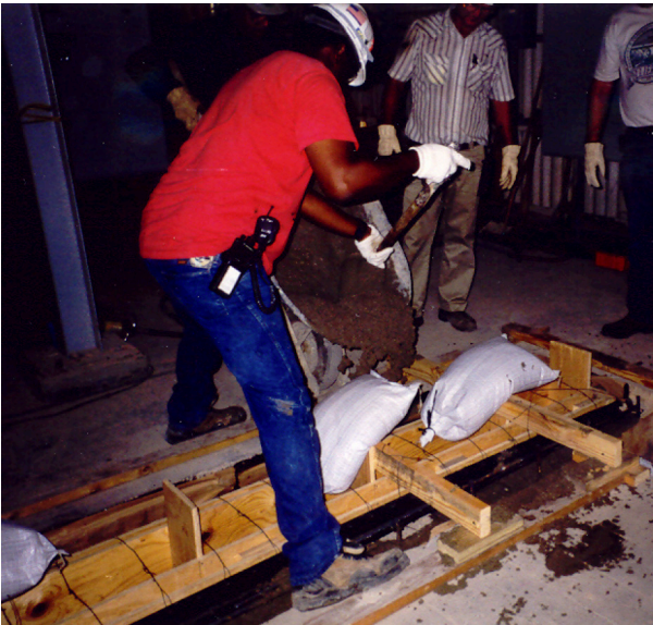
9. Workers shovel the first lift of Portland cement concrete (pea gravel mix) into the space between the trench and existing concrete.
